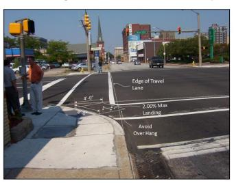
Diagonal ramps must have a 48"x48" landing area completely inside of the crosswalk and out of the travel lanes.
