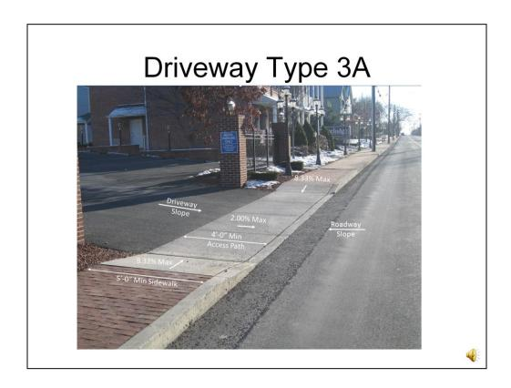
Type 3A driveways provide a moderate level of access. Here the sidewalk width is narrow and the sidewalk must ramp down to the depressed curb. This forces pedestrians to travel ramps and is not as ideal as other driveway types.
