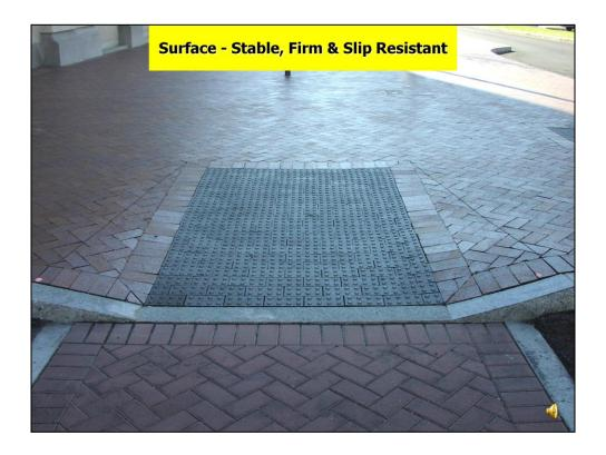
The surface of all facilities must be stable, firm and slip resistant. Grass is not a suitable surface. The picture depicts a curb ramp with truncated domes for the full depth of the curb ramp. This is no longer the requirement, but still compliant. Also depicted is a brick surface. When a brick surface is used, careful consideration must be used to avoid vertical lips as shown in the next slide.
