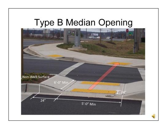
Type B Median Openings are very similar to Type A. Type B uses a 24" rolled flare. This is acceptable since it is not in the pedestrian path. Again, truncated domes are located on both sides to mark the travel lanes.
